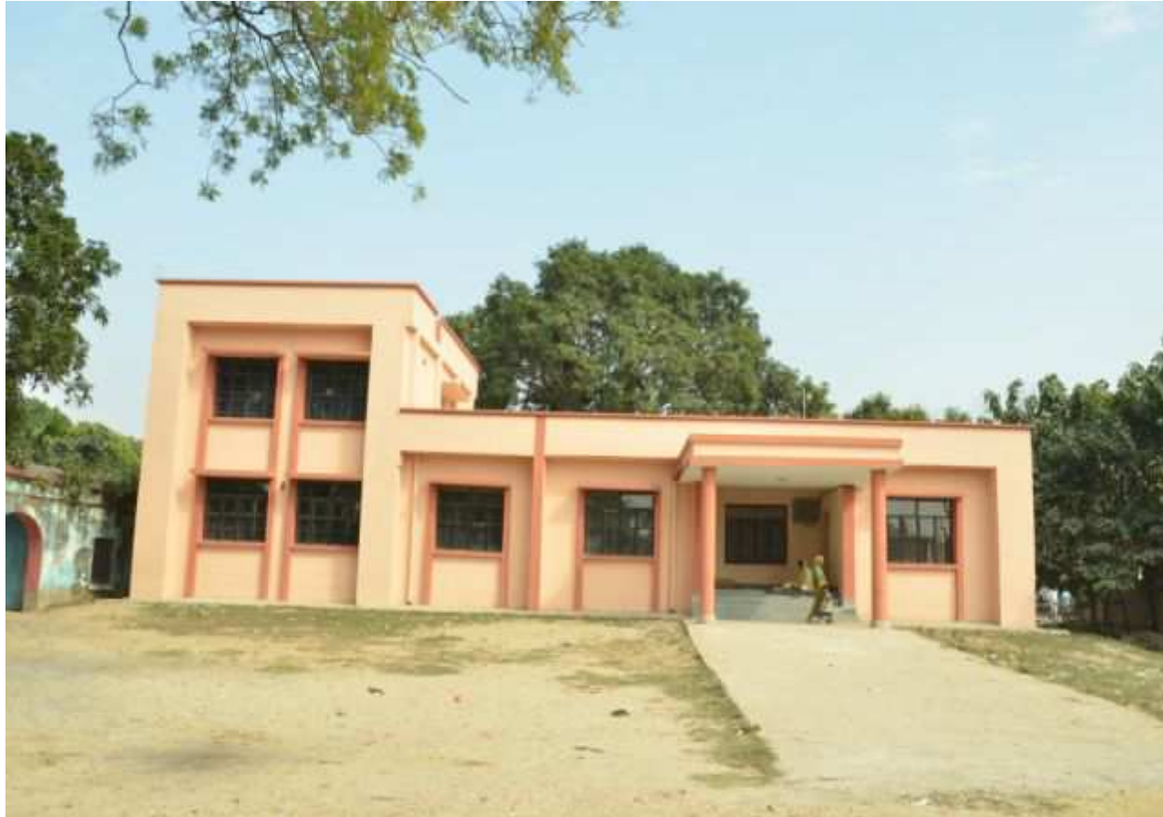
Sub Registry Office, Bahadurganj (Kishanganj)
