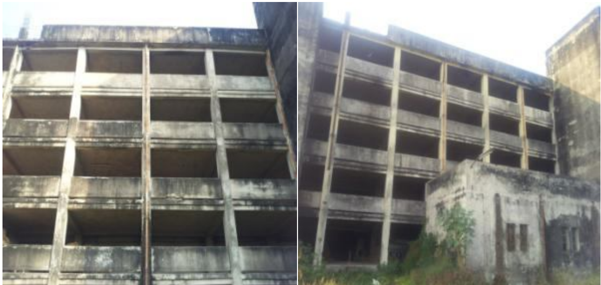
Photo plate: Project Site
